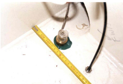
Accelerometer installed for onboard measurements
